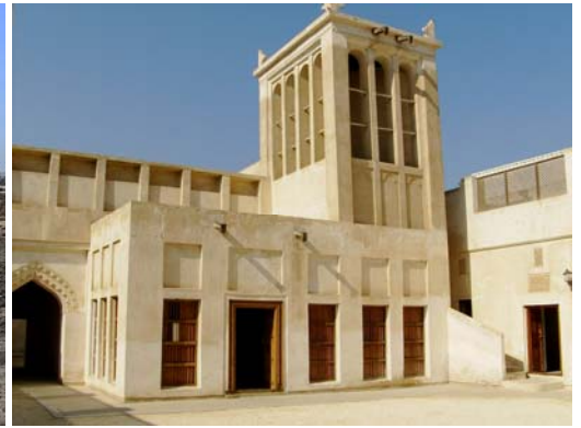
Windtower of Isa Bin Ali House, Pearling Path*
